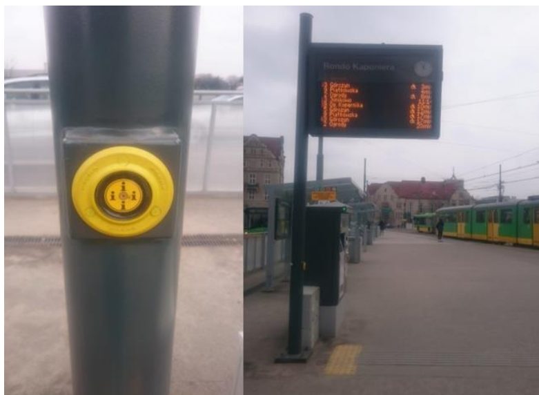
Fig. 9. Board with the time table at the stop Rondo Kaponiera. Push button, after pressing of which the time table is read aloud, is located at a height suitable for the requirements of disabled people; in front of the table a yellow warning texture is located and to the table itself blind people may be directed by the directing texture in the form of convex stripes on the ground (2018). Own elaboration
