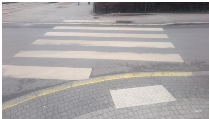
Fig. 11. Example of maladjusted pedestrian crossing in the public space in Poznań. Warning texture was not applied on the whole width of the crossing introducing a risk for blind people (2018). Own elaboration
