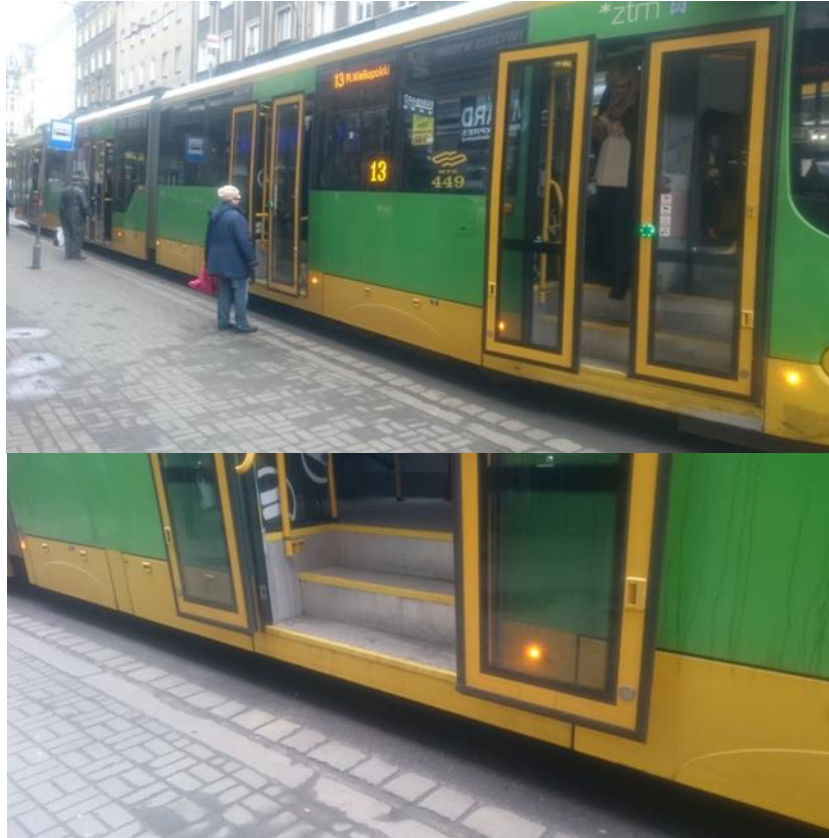
Fig. 10. East side of Gwarna street. Stop is maladjusted to the requirements of the user; lack of markings of the edge with yellow paint, lack of warning tabs for blind people, lack of elevation enabling ergonomic use of low-floor trams as well as the use of them by people on wheelchairs (2018). Own elaboration
