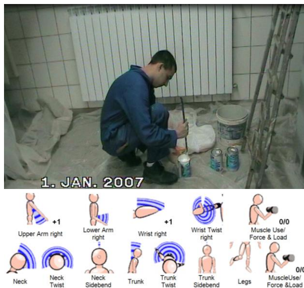
Rys. 7. Grand Score (right/left): 7/. A score of seven or more indicates investigation and changes are required immediately
